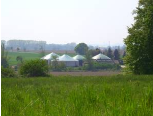
Biogasanlage in Lemgo © J.Dohmann 2007
